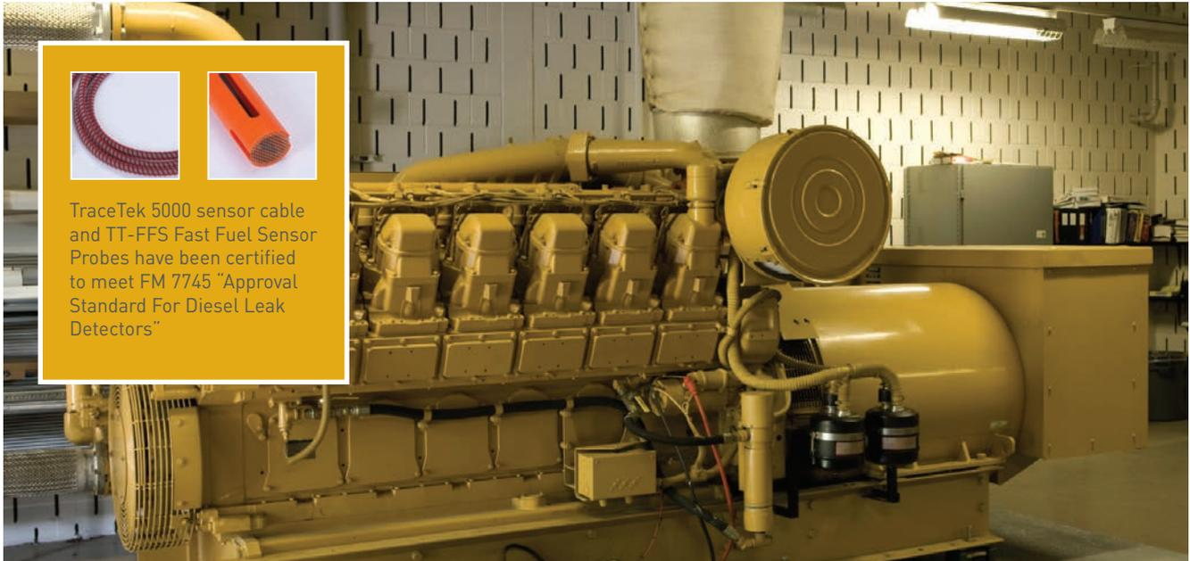
TraceTek 5000 sensor cable and TT-FFS Fast Fuel Sensor Probes have been certified to meet FM 7745 "Approval Standard For Diesel Leak Detectors"
